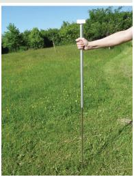
Installation of the fiberglass post with the **stake driver #49**
