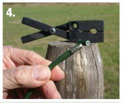
**4.** Bend the exposed wire back along the cable and insert into the connector
